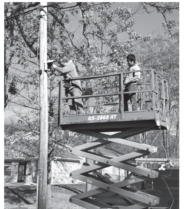
Ryan Dubie and Cory Dougan of Tandem Electric install newly rewired receptacles at a lower level on the light poles in the Village of Fruitport making it easier and safer for village workers to hang the lighted Christmas decorations
