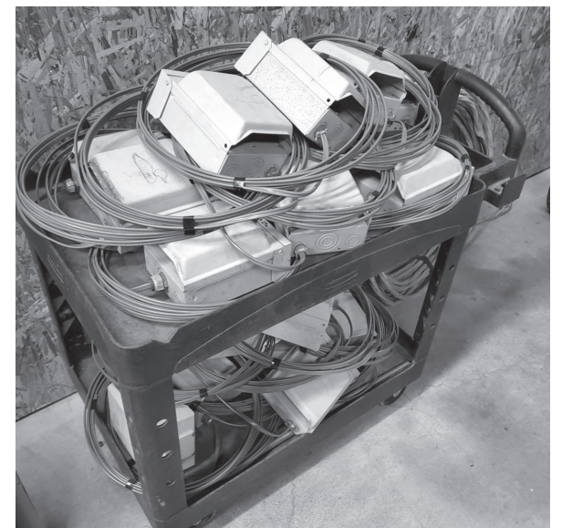
Newly rewired receptacles ready for installation
